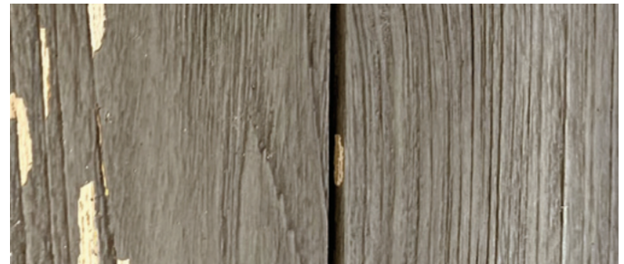
Partial weathering (some unpainted teak exposed)
